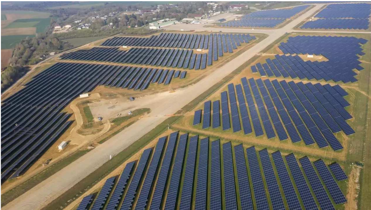
364000 solar modules over 155 ha in North of France (Meuse Dpt). 152 MWp capacity (23 000 hab)
