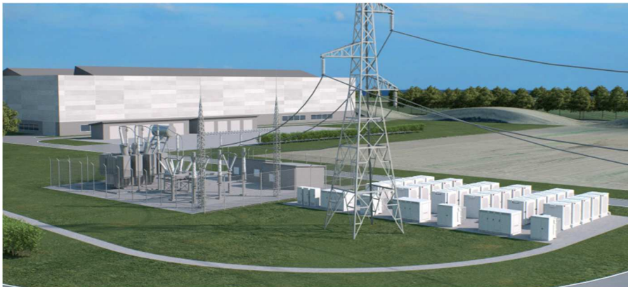
eStor-Lux (2021) - 10 MW/20MWh Li-ion battery storage station
