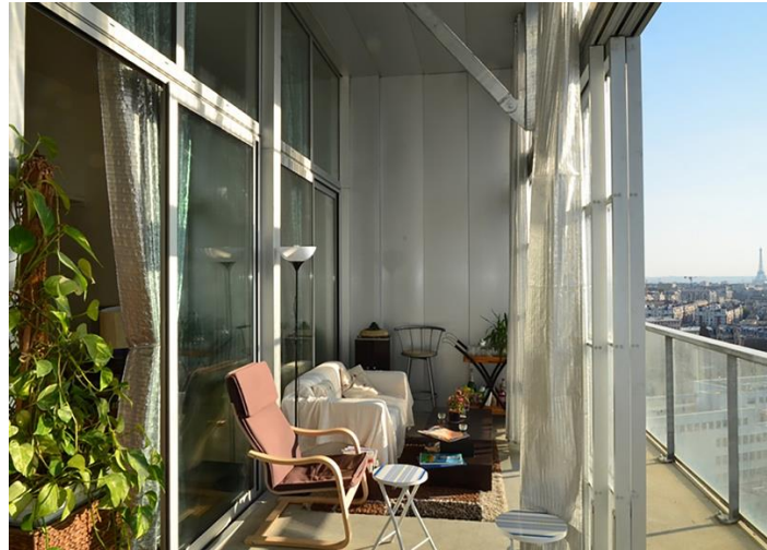
Figure 8. Frédéric Druot and Lacaton & Vassal revitalized Tour Bois-le-Prêtre (2011) in Paris, an apartment tower built in 1961, with an exterior of balconies and wintergardens along the exterior. (Photography: Frédéric Druot.)
