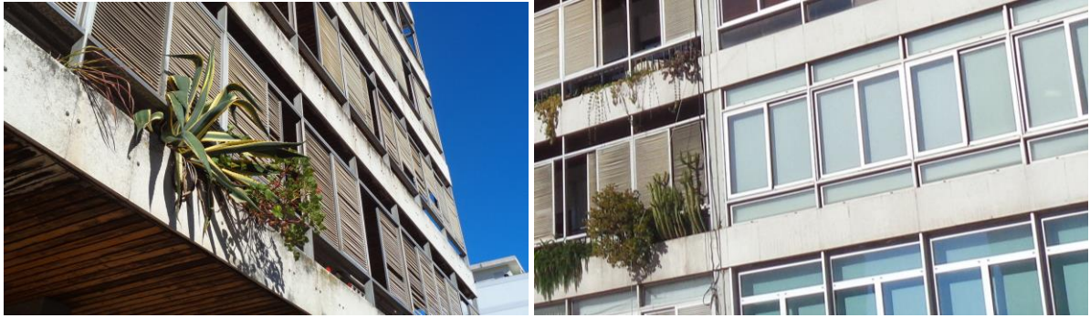
Figures 1 and 2. Open loggia (on the left) and glazed loggia (on the right)
