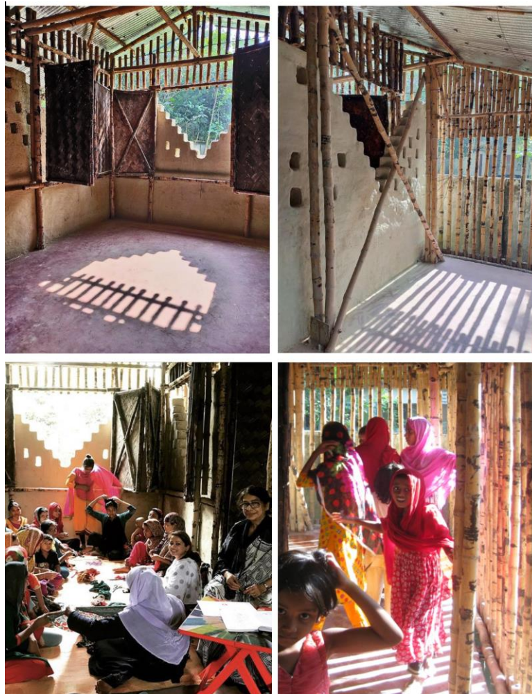
Figure 10. The Rajapur Women's Literacy and Community Healthcare Centre: The Rajapur Centre completed and being used by the community. Utilising evaporative cooling through its special perforated bamboo and earth walls as it hovers over the pukur, cooling the internal spaces.
