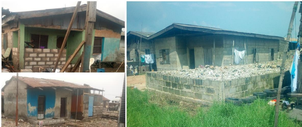
Figure 4. Reshaping existing building and higher floor for a new building.
