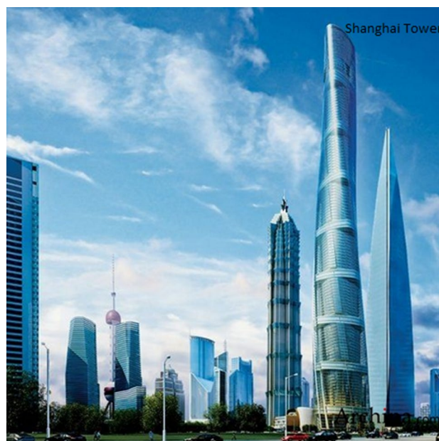
Fig. 2 Shanghai Tower and other Towers in Shanghai city (China)
