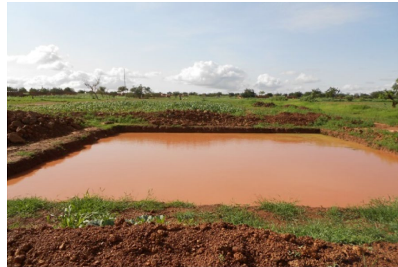
b) Pond with bottom and un-waterproofed walls on lateritic soil in Yatenga province
