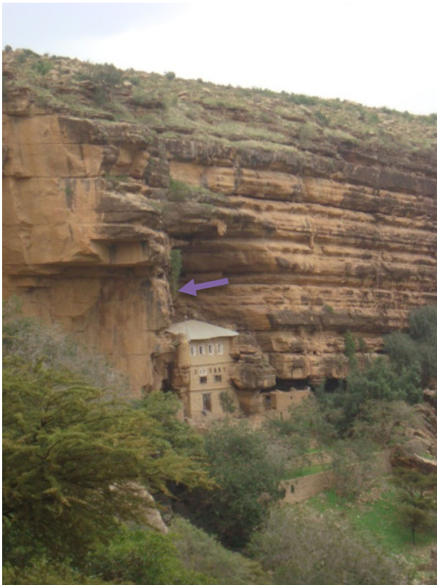
Fig. 1 The basal member of the Antalo limestone near Zeyi village. The Abune Aregawi church is built under the overhanging cliff that hosts a 364-m long cave in the limestone. Cave entrance is indicated by an arrow. Photo Jan Nyssen (2013). (Dramis and Fubelli 2019)
