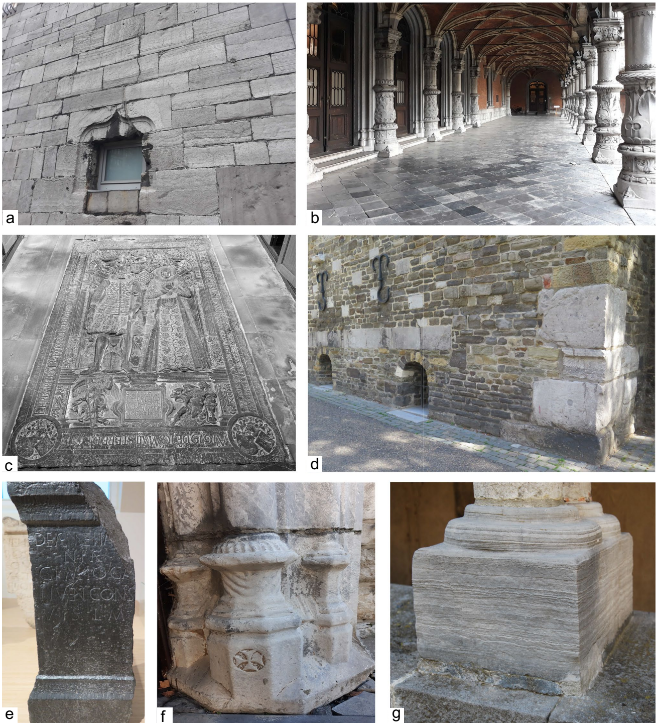
Fig. 7 Examples of use of the ‘Pierre de Meuse’. a Western wall of the fifteenth century cloister in stromatolitic facies, Saint Paul Cathedral, Liège. b Pavement of the courtyard of the Palais des Princes-Evêques, Liège in stromatolitic facies and ‘Marbre noir de Namur’. c seventeenth century incised tombstone in Schettens, Friesland, by P. Claes (courtesy of T. Brink). d Reuse of large Roman blocks of
