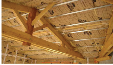
Figure 1.4: PCM installed on internal faces of a roof and a wall.
