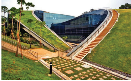
Figure 2.12: The green roofs at the School of Art, Design and Media, at the NanYang Technical University in Singapore.
