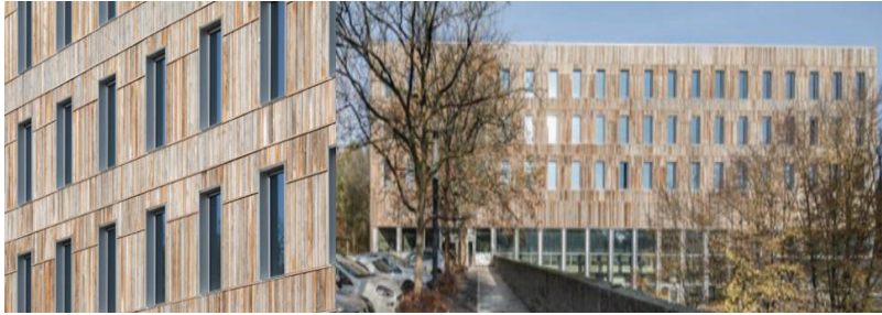
Figure 2.3: Institute of Botany at the University of Liège (Belgium) – facade renovation with reused wood (initial building: Roger Bastin, 1970; renovation: ULIEGE-ARI, 2018).
