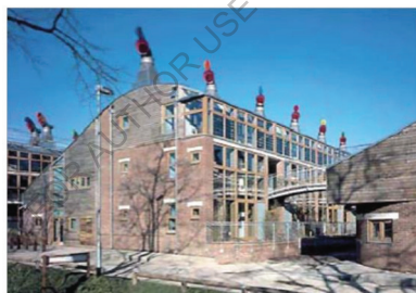
Figure 1.2: In BedZED neighbourhood, residential functions are oriented to the south, while the north facing parts of buildings are dedicated to tertiary functions.
