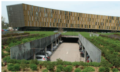
Figure 2.13: A green roof installed on a parking area in Linz (Austria).
