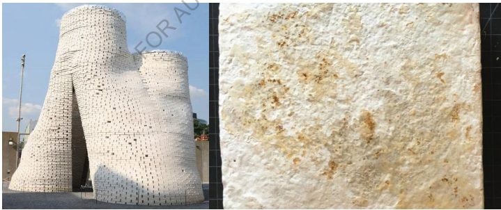
Figure 2.11: Mycelium used in a built structure.
