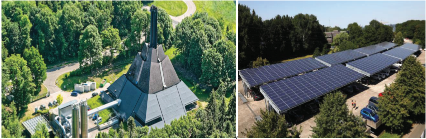
Figure 2.1: Biomass cogeneration unit of a district heating network (left) and renewable photovoltaic electricity production (right) at the Sart-Tilman campus of the University of Liège, Belgium.
