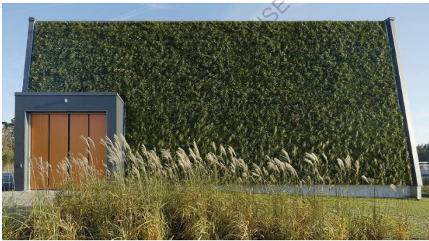
Figure 4.1: The new waste Envac vacuum system terminal in Stora Ursvik (Sweden), designed by Tengbom, is a BREEAM-certified industrial building. The collection station building is covered by a 250 m 2 green wall containing 2000 plants and over 20 varieties of grasses and herbs.
