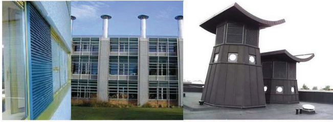
Figure 1.6: Intensive ventilation grid, integrated in an opening window (left), solar chimneys of the BRE building in UK (middle), and ventilation towers of the IVEG building in Belgium (right)
