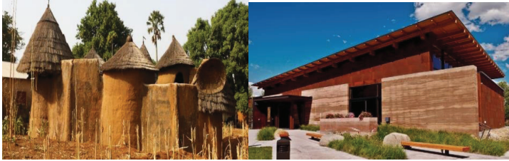
Figure 2.6: Buildings using rammed earth.
