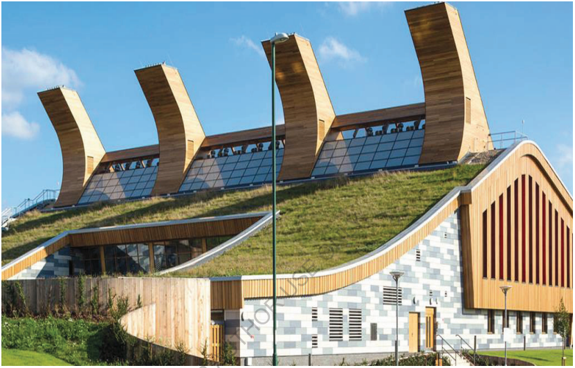
Carbon Neutral Laboratory, designed by Fairhursts Design Group, in Nottingham (UK)
