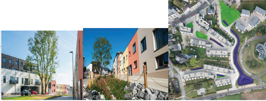
Figure 9.1: The studied eco-neighbourhood in Belgium, designed by FLW Architects.
