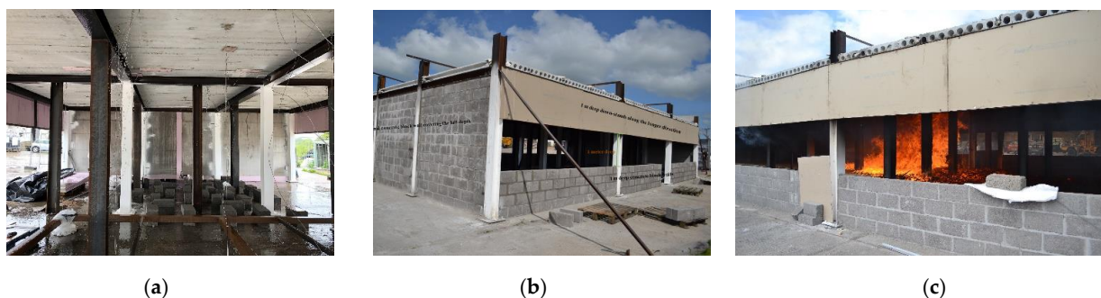
Figure 8. Photographs of the experimental campaign carried out by Ulster University in the frame of “TRAFIR” project: (a) steel frame with protected and unprotected columns; (b) compartment for test n°2; (c) fire at around mid-length of the compartment during test n°2.
