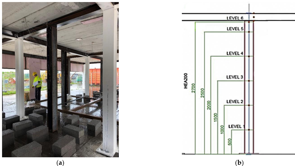
Figure 10. Photographs of the large scale natural fire tests carried out by Ulster University in the frame of “TRAFIR” project: (a) unprotected steel column with thermocouples; (b) levels of the thermocouples.
