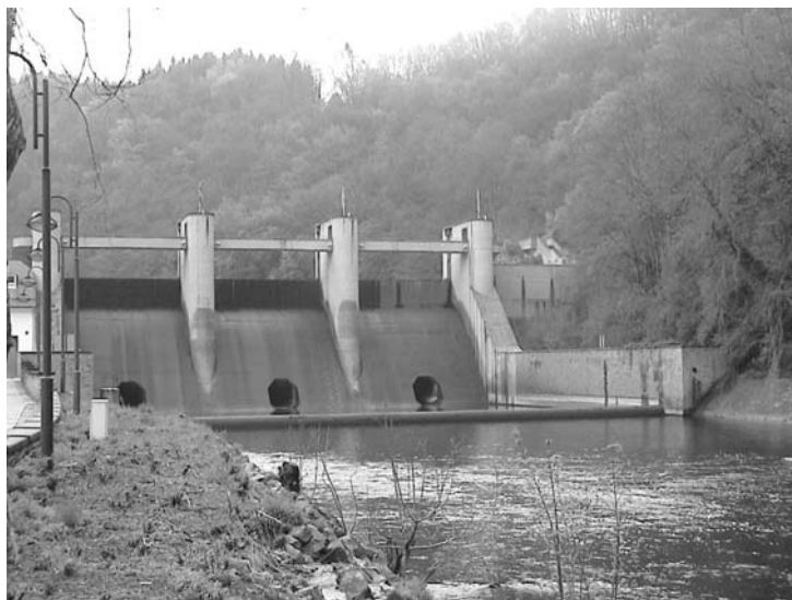
Figure 1: Nisramont concrete gravity dam
