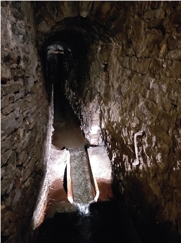
Figure 1. Mouth of the Richefontaine drainage gallery network, one of the four “ areines franches ,” just before entering the drinking water fountains. Photo by A. Anceau, 20 September 2020.
