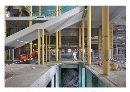
New railings and steel reinforcements superimposed onto the existing, 2021, ©Filip Dujardin
