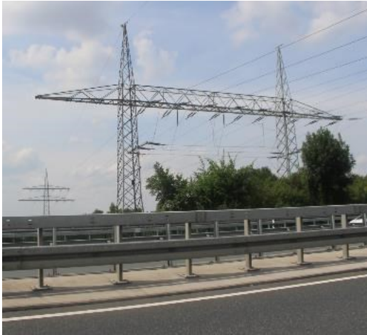
(a) Anchor portal tower
