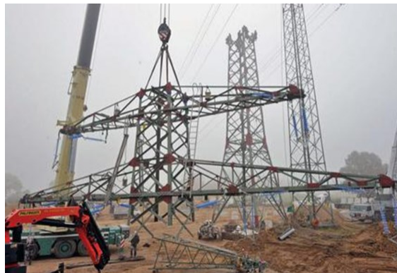
Figure 8.3: Modular construction with bolted connections.
