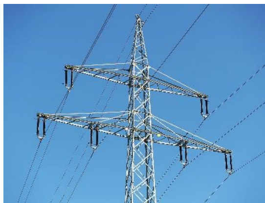
Figure 8.7: Cross arms of a lattice tower
