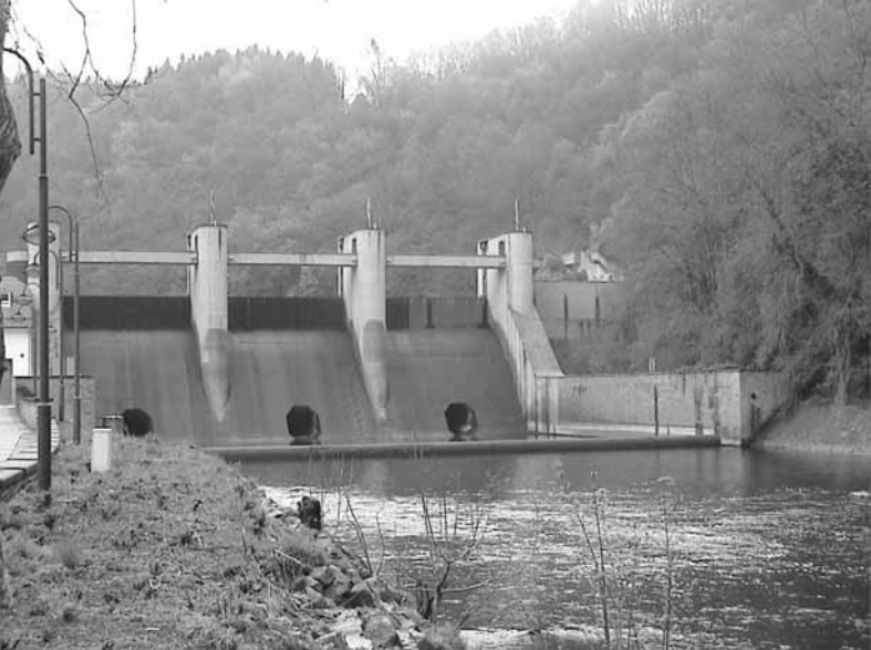
Fig. 1 Downstream view of the Nisramont dam © HACH
