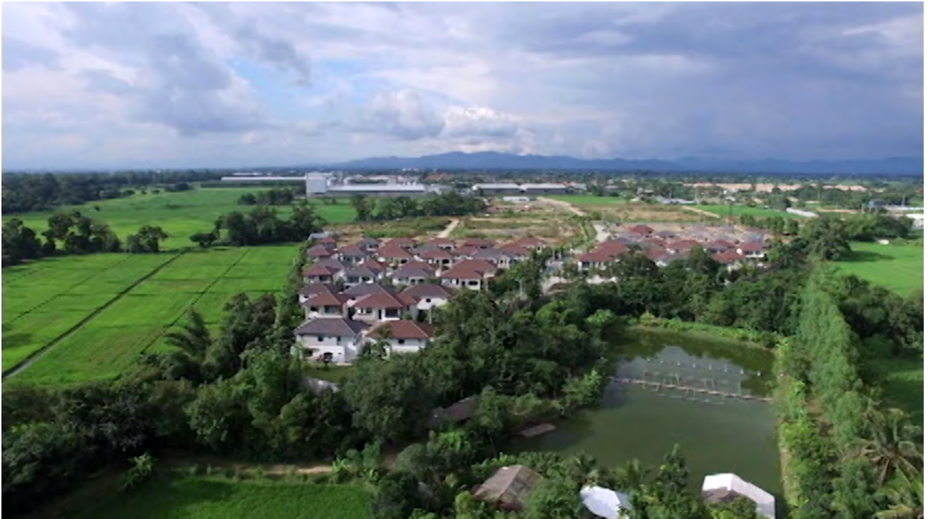
Figure 10. A high wall separates rice paddies and fish ponds from new gated community under construction within the agricultural preservation zone east of the Kuang River. Industrial food processing sheds can be seen in the background. Drone imagery: Santipab Sonboom, October 2016.
