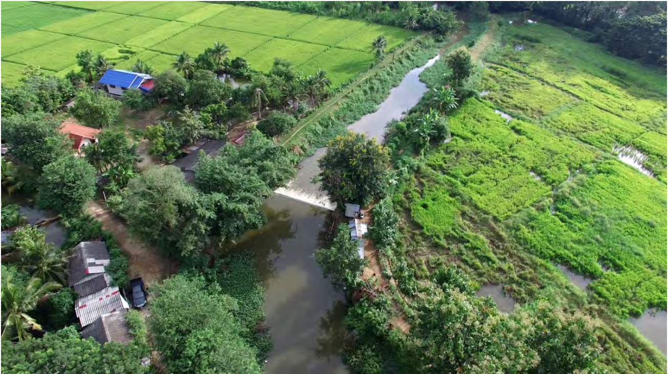
Figure 4. Muang (canal) fai (weir) on the Kuang River inside Chiang Mai’s outer ring road. The weir in the center of the image creates a retention pond at a higher level that supplies the canal on the left of the frame, which in turn gravity-feeds the rice paddies in the upper left of the frame. The cultivated rice paddies on the left are on the east side of the Kuang River within the agricultural protection zone, however the ring road is just out of the frame to the left. The unmaintained paddy on the right is within the low-density housing zone west of the river. Drone imagery Santipab Sonboom, October 2016.
