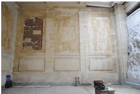
Interior view, decorative marble panels before restoration, 2012*.
