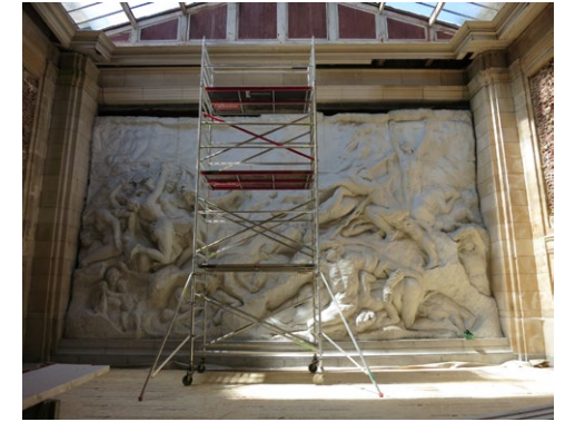
Interior view, during restoration*.
