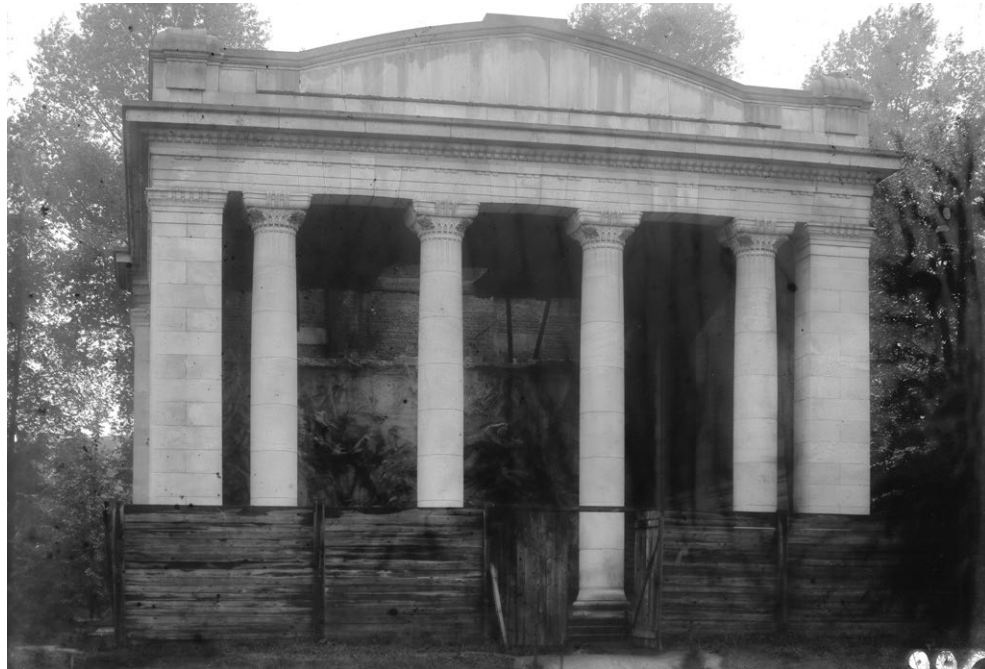
The Pavilion of Human Passions, arch. Victor Horta, 1904-1905. A wooden barricade has been built to prevent access to the building. The roof lantern is obscured so that light can only enter through a central opening directly above the relief. (© Belgian Buildings Agency - Ministry of Public Works Fund)
