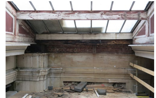
Interior view of the glass roof during restoration work, 2013*.
