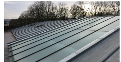
View of the roof after restoration work, 2014*.
