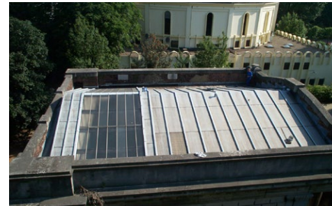
View of the roof prior to restoration work, 2002*.
