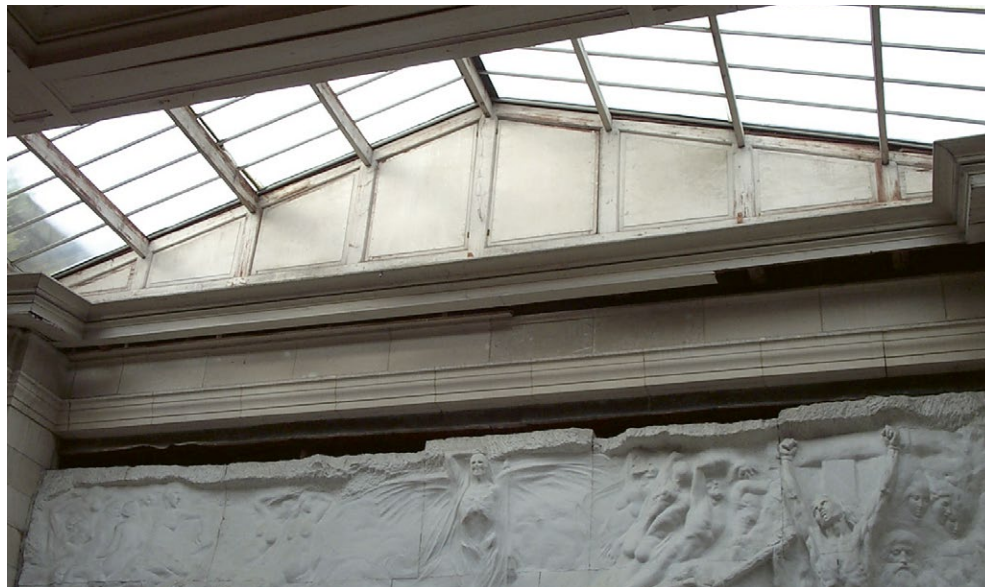
The Pavilion of Human Passions, arch. Victor Horta. View of the relief before restoration: the Euville limestone edging at the top is missing, having been taken down in 1980 (photograph taken in 2003). (© Belgian Buildings Agency)
