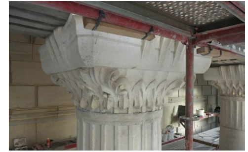
Euville limestone capital after restoration, 2014*.
