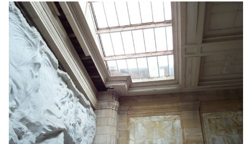
Interior view of the glass roof prior to restoration work, 2002*.
