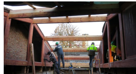
Dismantling of the glass roof during restoration work, 2013*.
