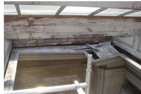
Interior view of the glass roof prior to restoration work, 2005*.
