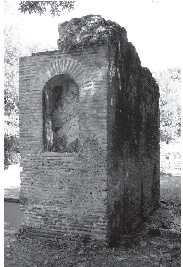
54. View of the south side of the apse, with flat niches.
