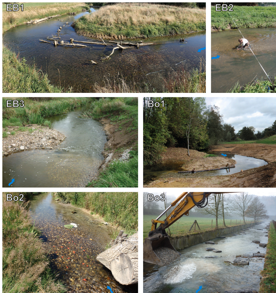
Fig. 2. Spawning study sites. Gravel was arranged along hydraulic structures made of wood at sites EB1, Bo1 and Bo2 and upstream of rock weirs at site Bo3. Sites EB2 and EB3 have no hydraulic structures. The PIT-tagged gravels are visible in red at site Bo2. (For interpretation of the references to colour in this figure legend, the reader is referred to the web version of this article.)
