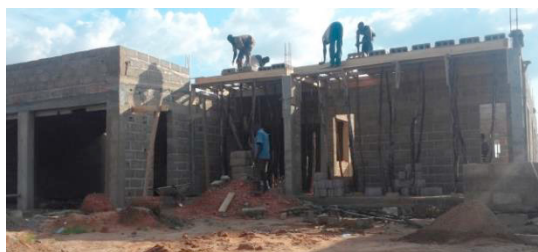
Fig.1 Construction of cement blocks dwelling in Ouagadougou
