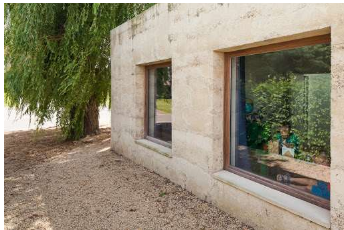
Fig. 11 Rammed concrete wall [27]
