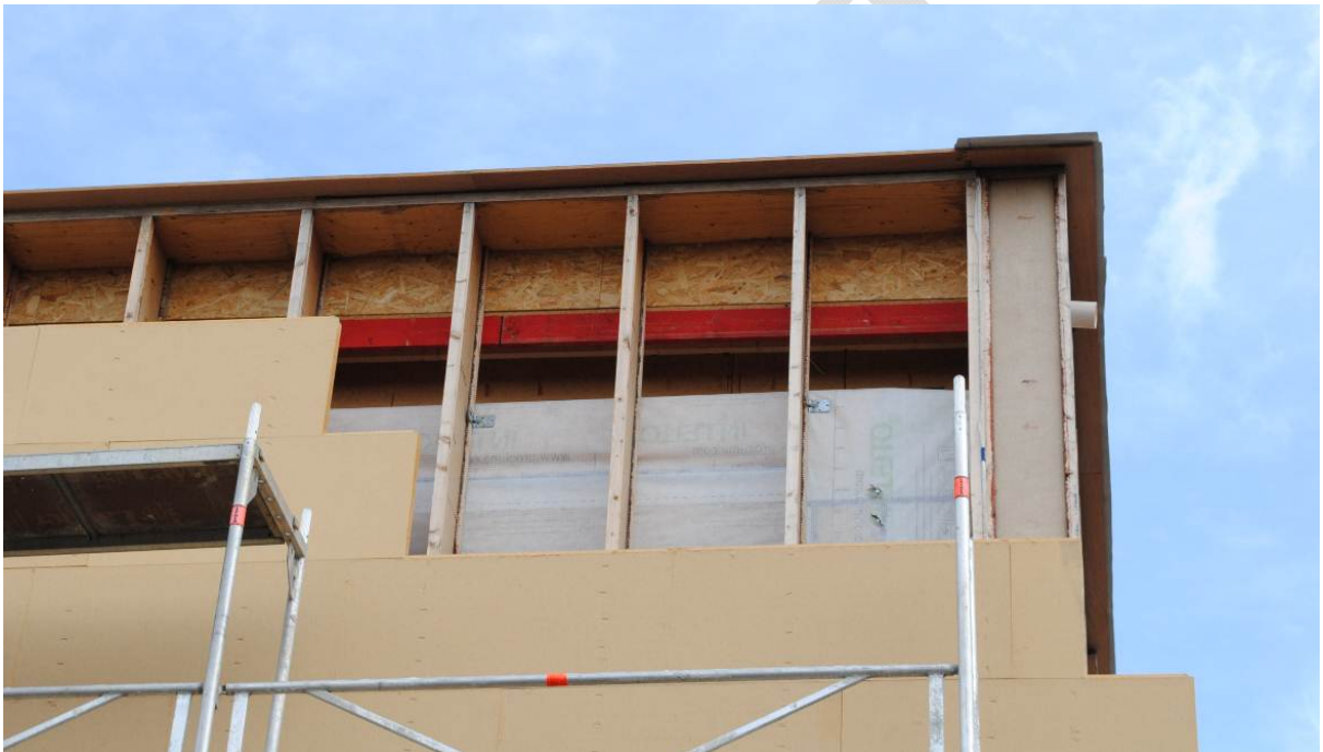
Figure 4: Composition of the external wall
