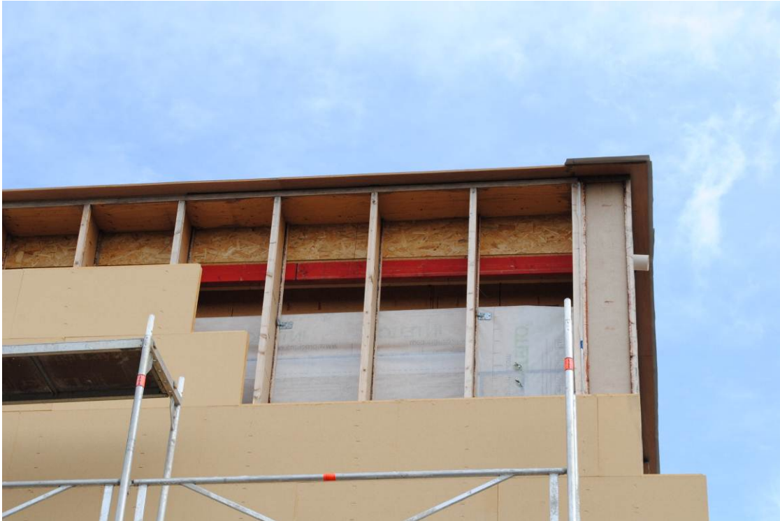
Figure 1: Boxes before the insulation
