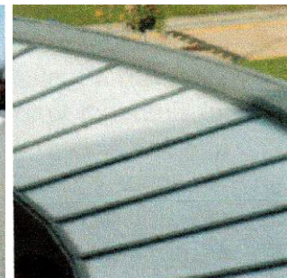
Systeme of skylights of polycarbonate
