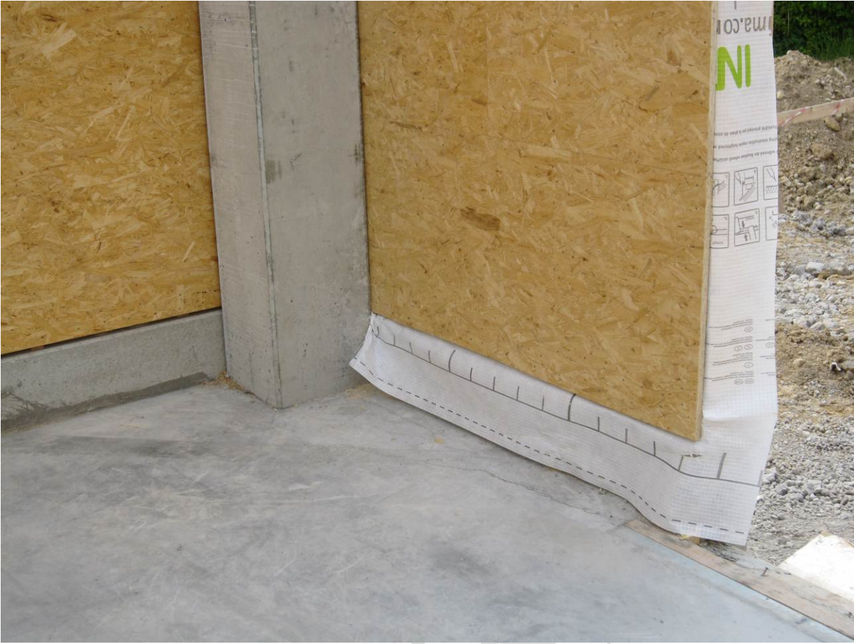
Figure 7. Detail of the structure
