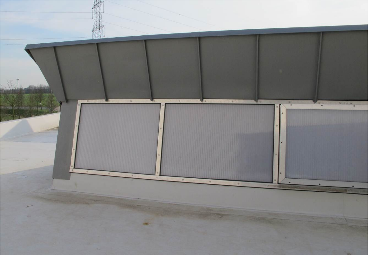
Figure 2. Outside view from the skylight
