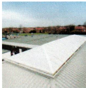
Skylights , light shaft and releases of smoke
