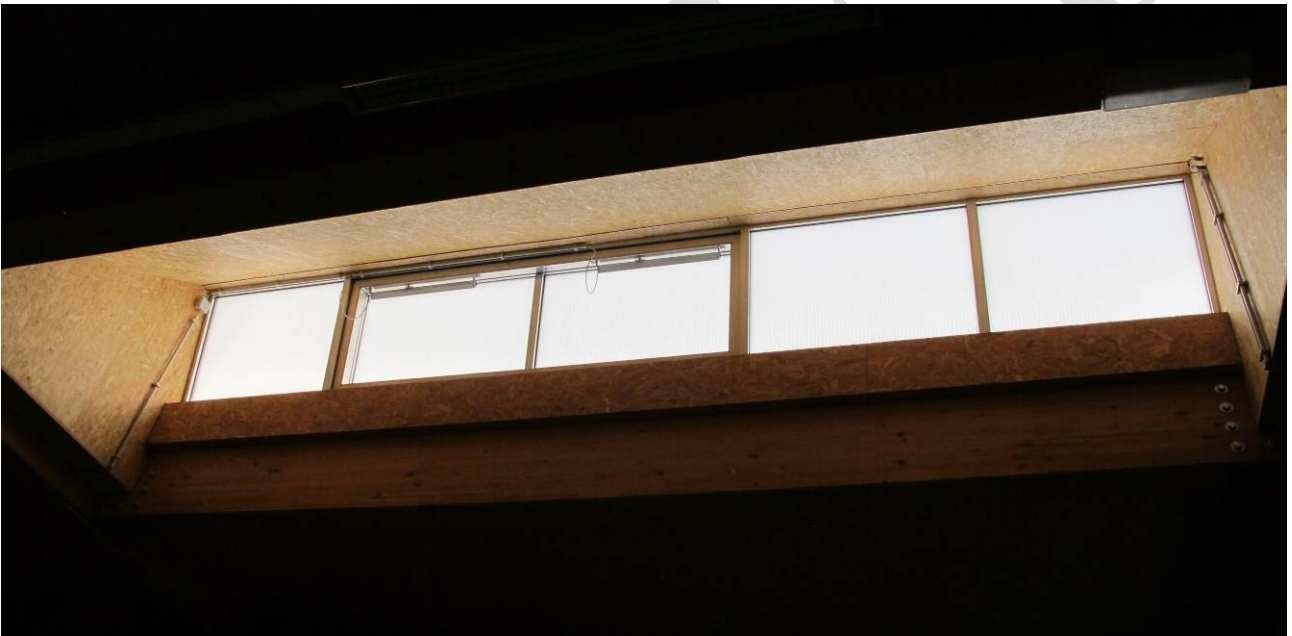
Figure 1. Inside view from the skylight
