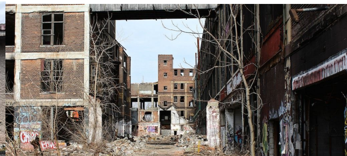
Packard plant, Detroit
