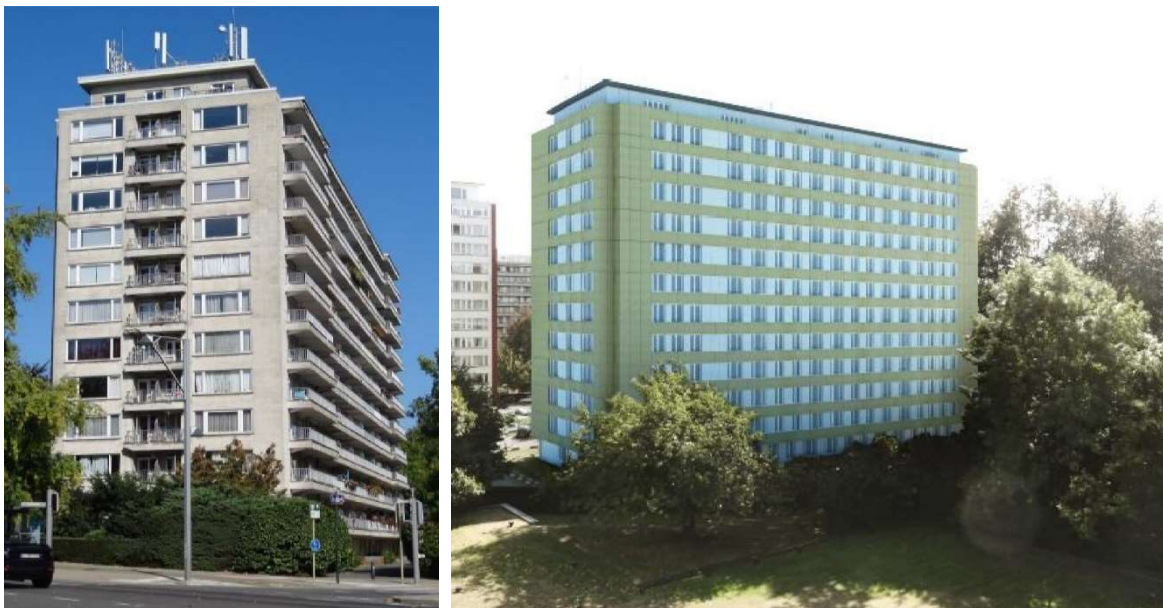
Fig. 1: The Expo I condominium in Jette (Brussels), before (left) and after (right) retrofit
