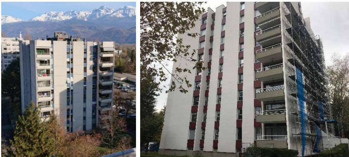
Fig. 1: The Manival condominium in Grenoble, before (left) and after (right) retrofit
