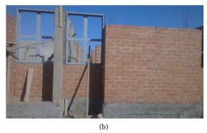
**Figure 1.** Construction of house whose walls are made of earth bricks: (a) Adobe brick with cladding, (b) CEB, Ouagadougou, Burkina Faso.
