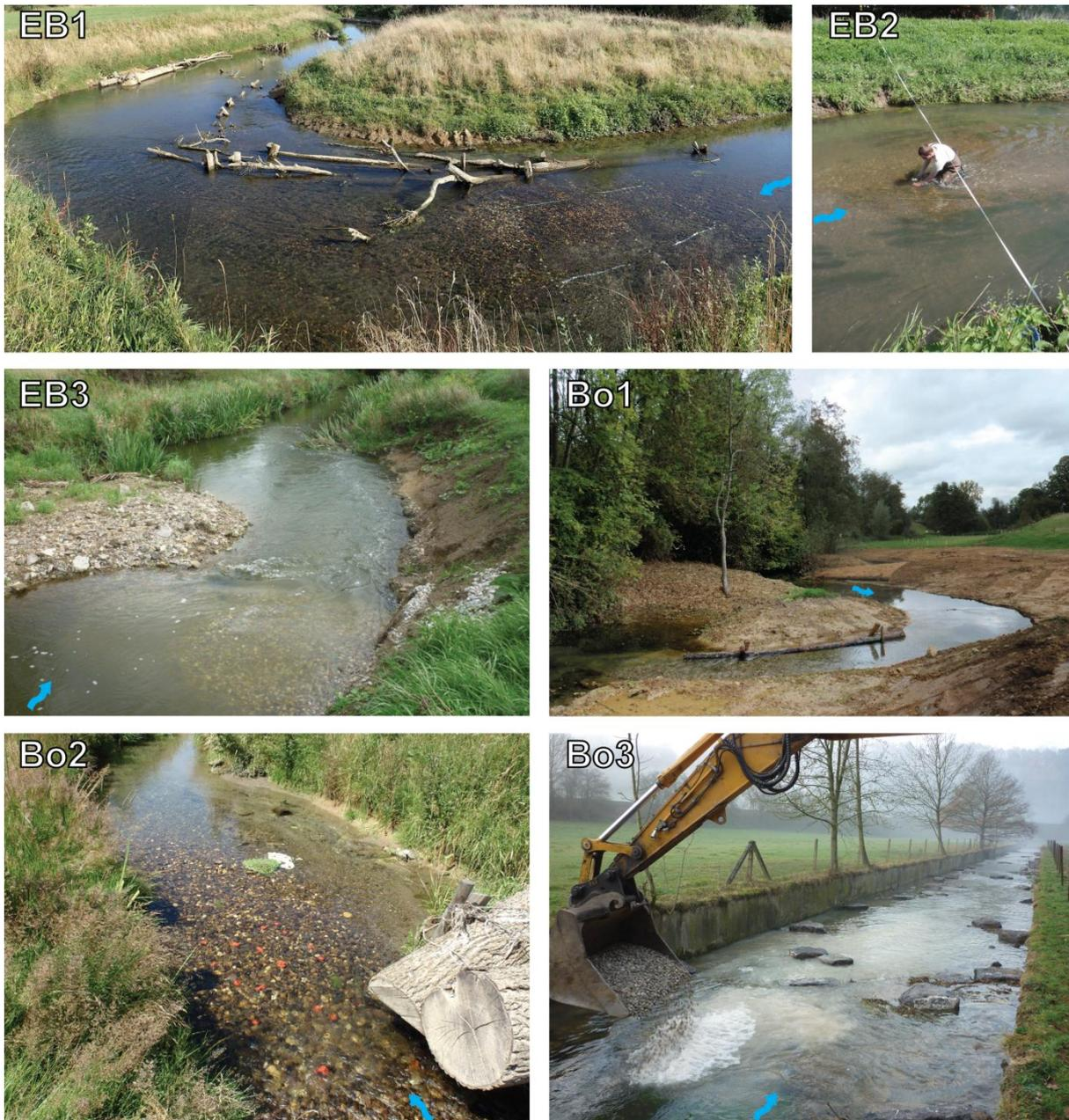
Figure 4.2 : Spawning study sites. Gravel was arranged along hydraulic structures made of wood at sites EB1, Bo1 and Bo2 and upstream of rock weirs at site Bo3. Sites EB2 and EB3 have no hydraulic structures. The PIT-tagged gravels are visible in red at site Bo2.
