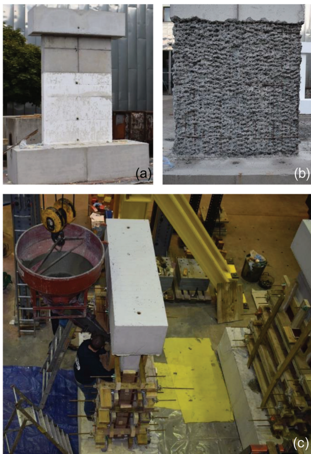
Fig. 4—Construction of test specimens.
