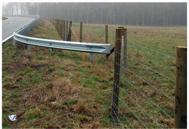
Figure 4 – fence placed along the N88 in Meix-devant-Virton, more than 300 km of this type of fence were placed to confine the boars and facilitate destruction
