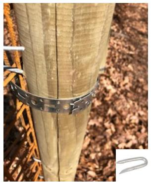
Figure 5 – Attachment of the panel to the stake using jumper nails and perforated tape
