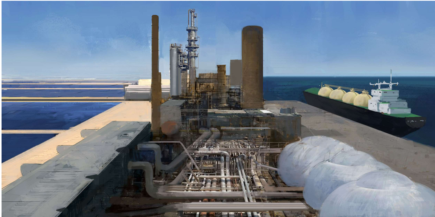
Artist representation of an infrastructure where solar energy and direct capture of \text{CO}_2 in the air are used to produce green \text{CH}_4 . The green gas is then liquefied and shipped to consumption centers.
