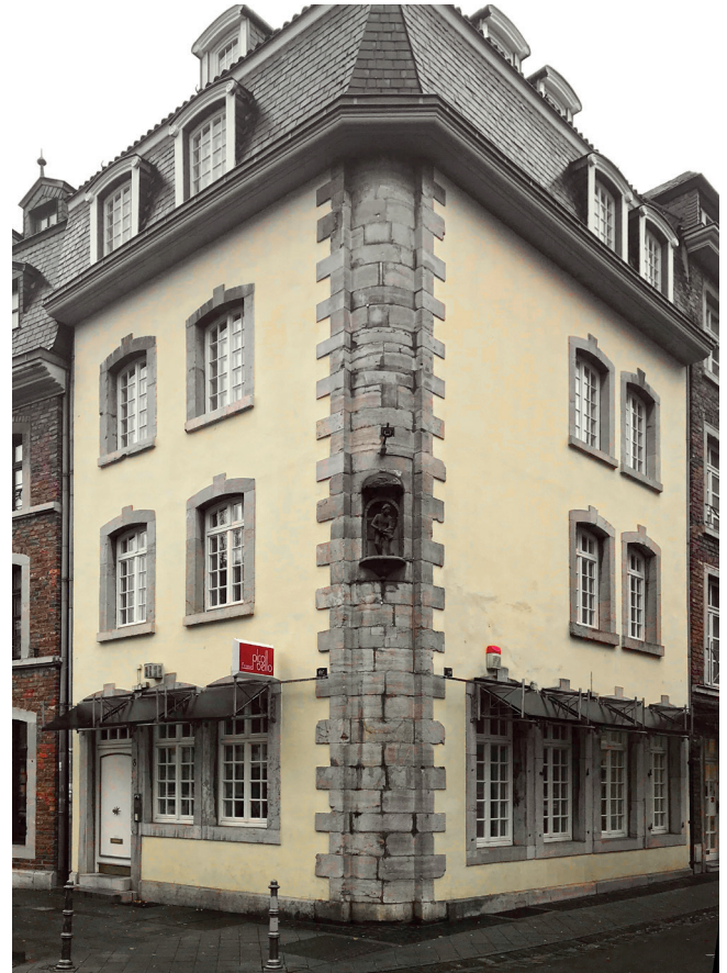
Fig. 0.9. Aachen Neupforte 8. Rebuilt house of 1980, Composed of parts of at least three maybe four different buildings stored at the building yard (©Jan Richarz).
