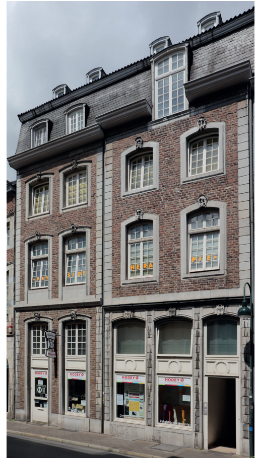
Fig. 0.7. Aachen Jakobstraße 14-16. Two of three facades dismantled in 1965 about 300 m away in Großkölnstraße to be stored for further use. After some consideration all three were used in the same alignment as before and missing parts were added, located in redevelopment area 1. (©Jan Richarz)
