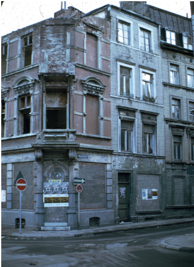
Fig. 0.8. Aachen Neupforte 8. Ruin of the war around 1975, the neighbouring houses with bricked up doors and windows (©Leo Hugot).
