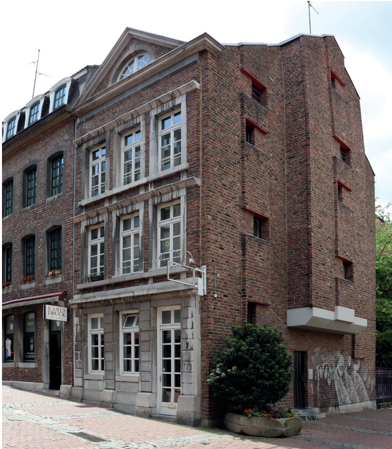
Fig. 0.6. Aachen, Kockerellstraße 9. Originally located at Peterstraße 47, this facade was torn down in 1963 and stored until 1974 when it was relocated to its new site within the redevelopment area 1. No changes were made in its arrangement. As can be seen here, the other facade around the corner looks decidedly modern. (©Jan Richarz)
