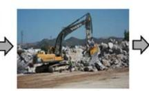
3. Initial processing (crushing, separation, etc.)
