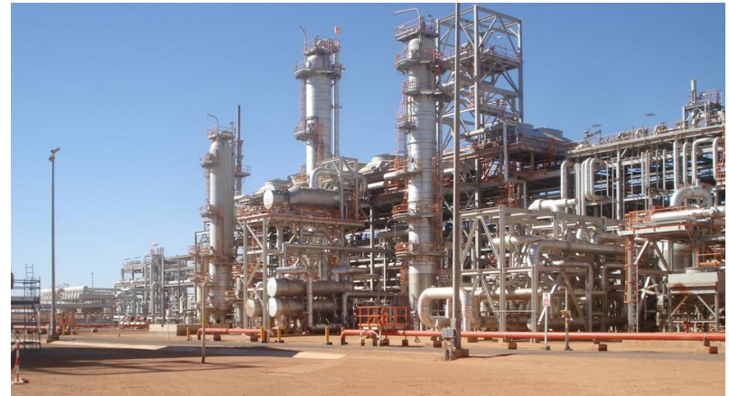
Algeria, Natural gas sweetening: 1400 -2800 tpd CO 2
