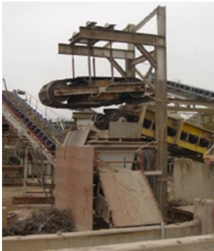
Figure 15 : electromagnet band for extracting steel
