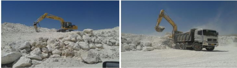
Figure 23: Gypsum extraction plant (“Photo Gallery,” n.d.)
