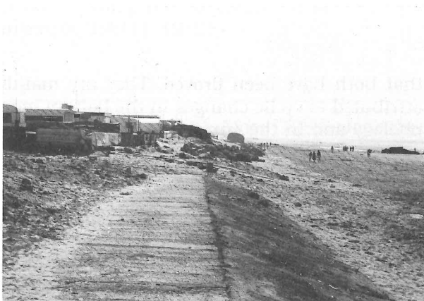
Plate 50-4. De Panne (1980). French-Belgian border. World War II blockhouses left on the present-day forebeach after dune retreat due to the local strike of an erosive mega-protruberance (photo by G. De Moor).
