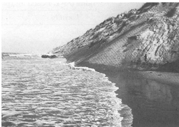
Plate 50-3. Klemskerke (1978). Effects of erosive megaprotuberance. Concrete dike built in 1910 against past sand waves, afterward completely covered by dune accretion and progression and since 1978 exhumed from underneath the dunes by the present-day retreat of the dune foot due to the repeated erosive action of sand waves (photo by G. De Moor).
