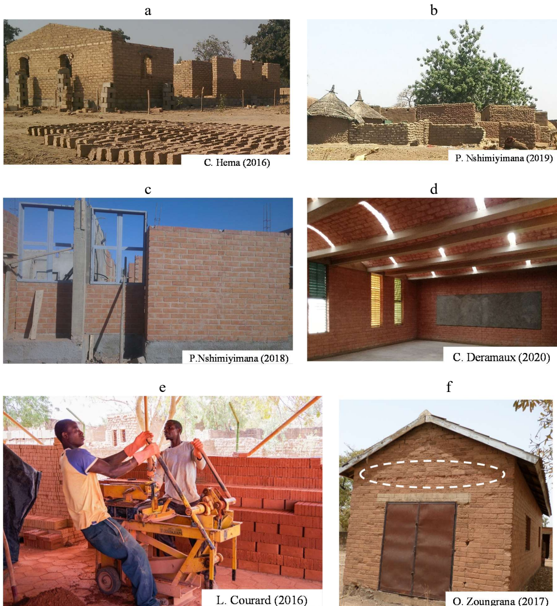
Figure 0.3. Earth in contemporary constructions, in the vicinity of Ouagadougou: low quality of adobe (a) construction site, (b) Wemtenga village versus improved quality of CEBs (c) construction site of a health center in Ouaga2000, (d) inside the Wemtenga primary school, (e) production of cement-stabilized CEBs at local enterprise, (f) erodability of a house in Kamboinse
