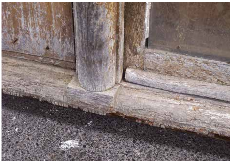
Fig. 10.13. Ancient abbey of Saint-Pierre-sur-Dives (department of Calvados): detail of the window sill and weather boards in quarter round form.
