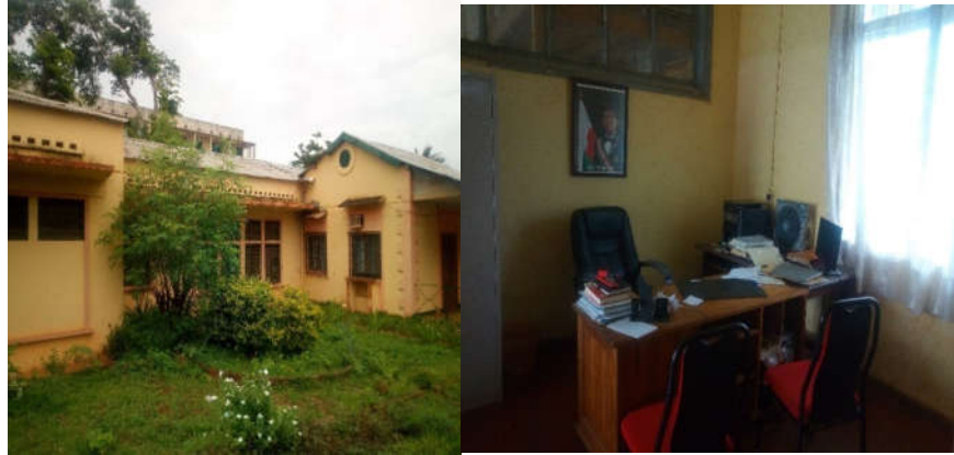
Figure 2. East facade of the studied office building.
