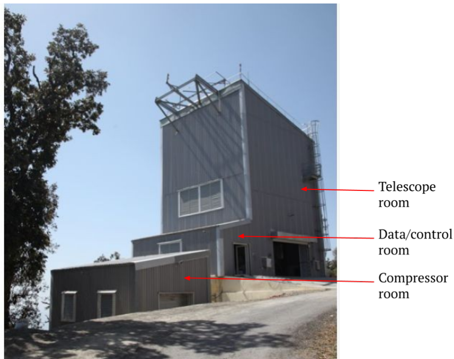
Figure 5.1: View of the ILMT telescope room, data/control room and compressor room.
