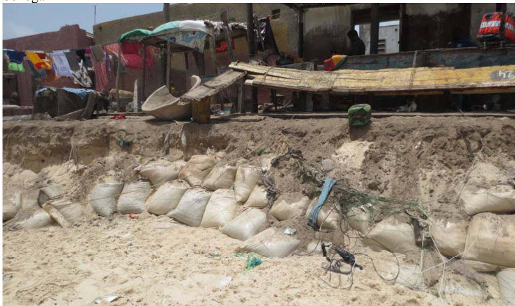
Figure 2: Sand bag barriers stabilized with old fish netting. Goxum Bacc, Saint-Louis, Senegal
