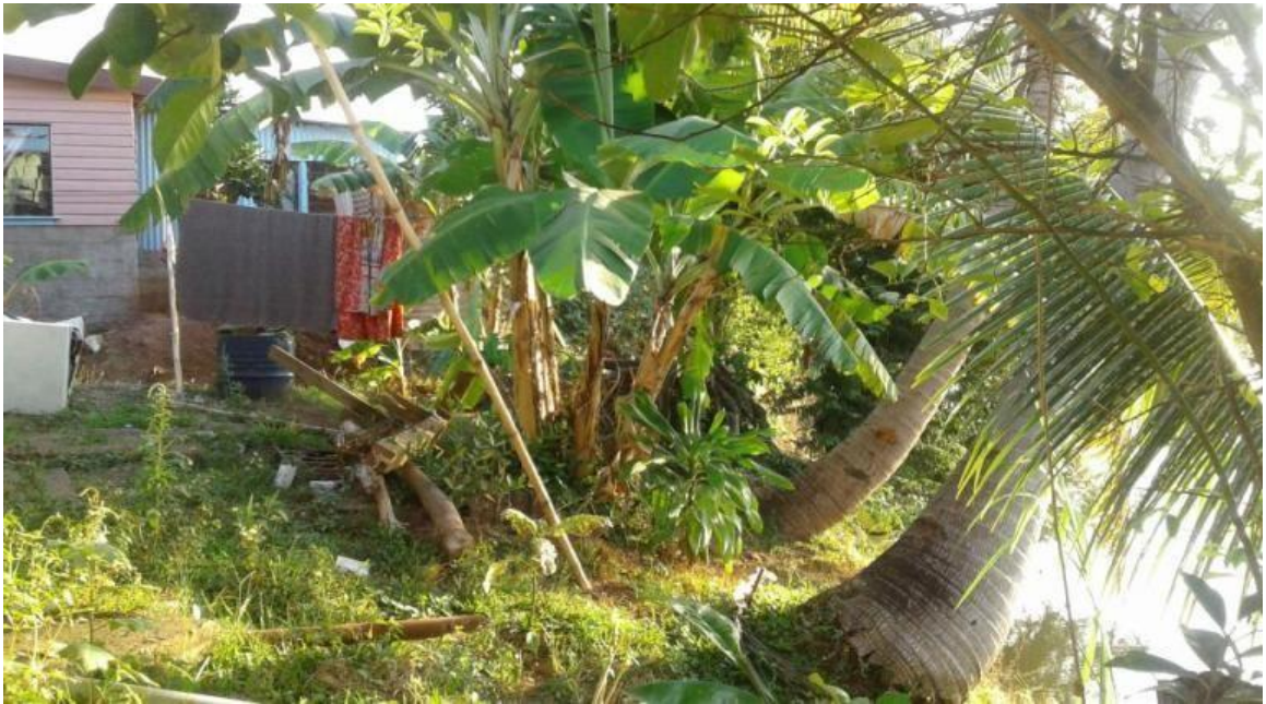
Figure 55: Palm trees described by Matawalu villagers as « seawalls » protecting their homes from flooding by the nearby river. Piles of wood are also regularly added by the community to protect their homes (Photo: Dalila Gharbaoui).
