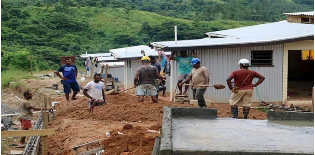
Figure 62: Men at work in the new construction site. (Photo: Julie Cleaver/PMC)
