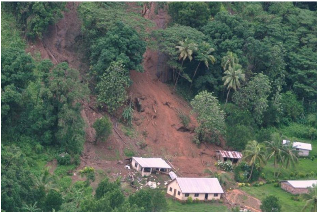
Figure 48: Destructive landslides in Tukuraki Village (Photo: Janet Lotawa).
