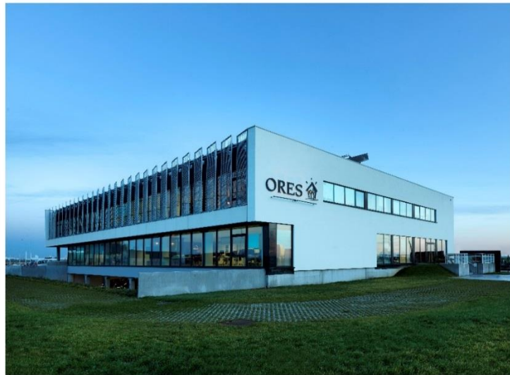
Illustration 4 - New building of ORES WaPi, in Leuze-en-Hainaut (source: ORES; permission granted by ORES)
