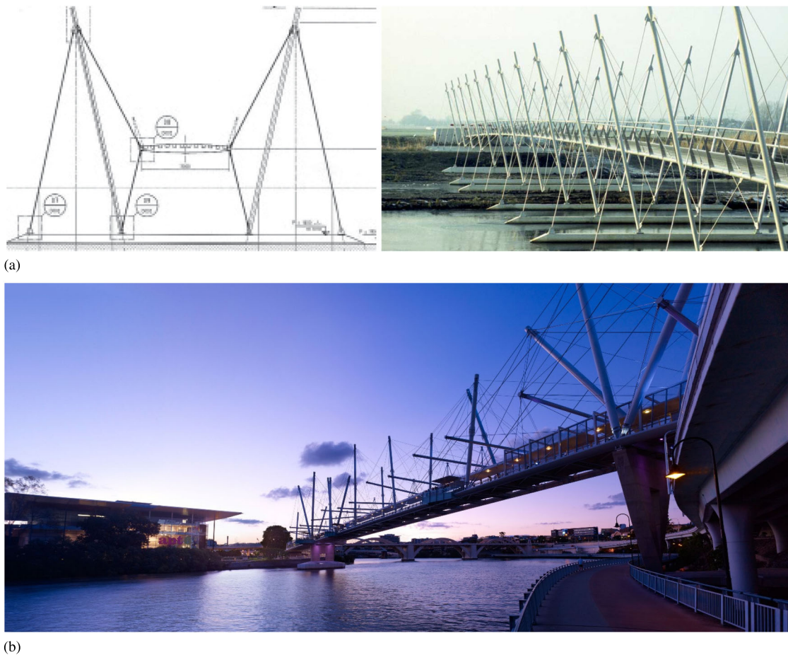
Fig. 2. Existing footbridges: (a) Bridge of Masts (2000, Purmerend, Netherlands) by den Hollander (reprinted from Eekhout 2016, with permission); and (b) Kurilpa Bridge (2009, Brisbane, Australia) by Cox Rayner Architects and Arup (Image credit: redbrickstock.com/Alamy Stock Photo).
