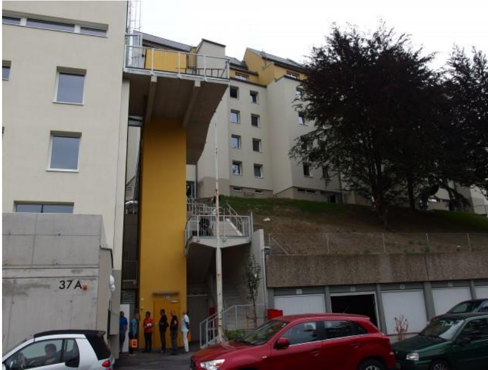
Figure 1-5: Stairs and elevator (colored in yellow) constructed specifically for the added floors on the rooftop in Kierling, Austria © Georg Reinberg
