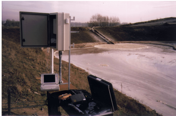
Settling ponds of sugar factories
