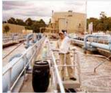
Waste water treatment ( sludge stabilization )
