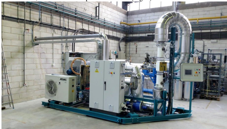
Fig. 2. Dual cell convective dryer using either air or superheated steam
