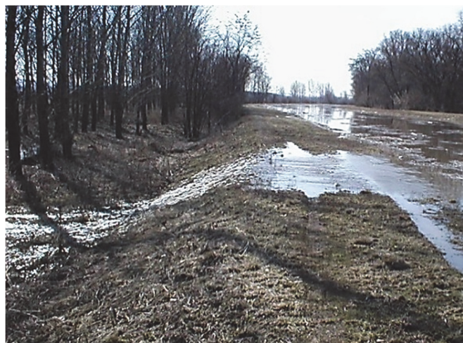
Fig. 1. Levee overtopping, to some extent similar to the flow over a broad-crested weir.
