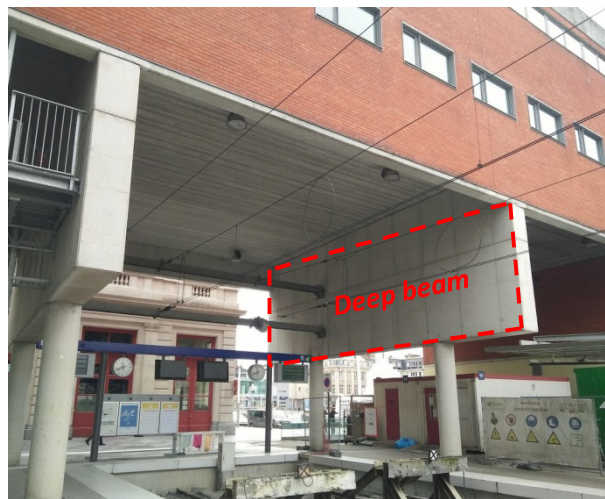
Fig. 1.2 Deep transfer girders in the train station of Leuven, Belgium
