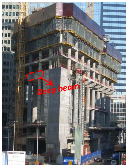
(a) During Construction
