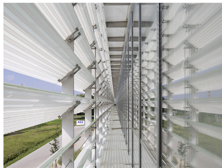
Figure 3. (Left), overview of the façade with the automated louvers opened; Fig. 3 (right) Exterior – Windows Double-skin façade combining glass louvers made of extraclear glass (outside skin) with super-insulating glazing and white spandrel double glazing (inside skin); Architect: Philippe SAMYN and PARTNERS sprl, architects and engineers – BEAI sa, Photographer: Jean-Michel Byl, Courtesy Notice: AGC Glass Building - © Project: Philippe SAMYN and PARTNERS sprl, architects and engineers – BEAI sa [33].
