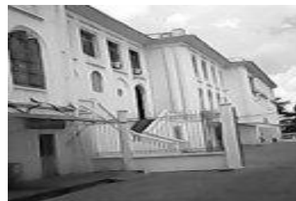
Figure 2 - Example of modern buildings studied.
