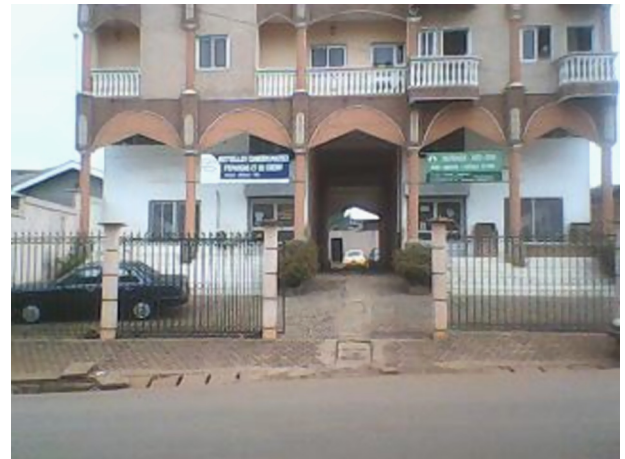
Fig. 2. Example of analyzed modern style building made by brick.
