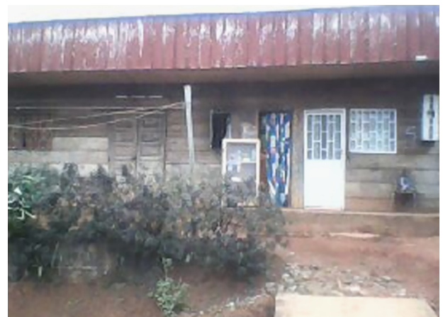
Fig. 3. Example of analyzed traditional style building made by board.
