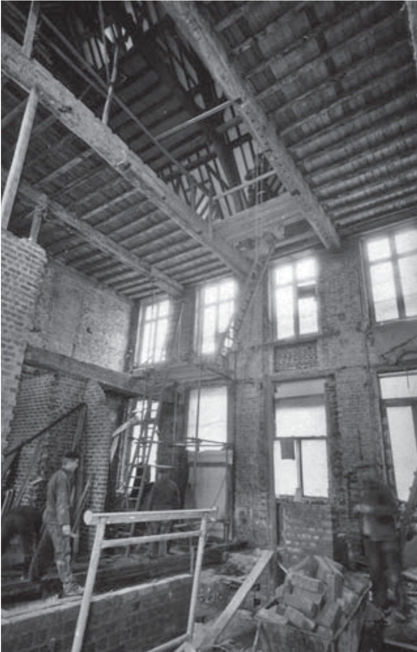
33/n. 92, interior view during the works, 1967 (ARML).
